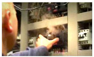
Figure 3 Preben pulling out a smoking controller out the control cabinet
