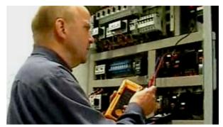
Figure 4 Preben using a volt meter to measure electric current in the control cabinet
